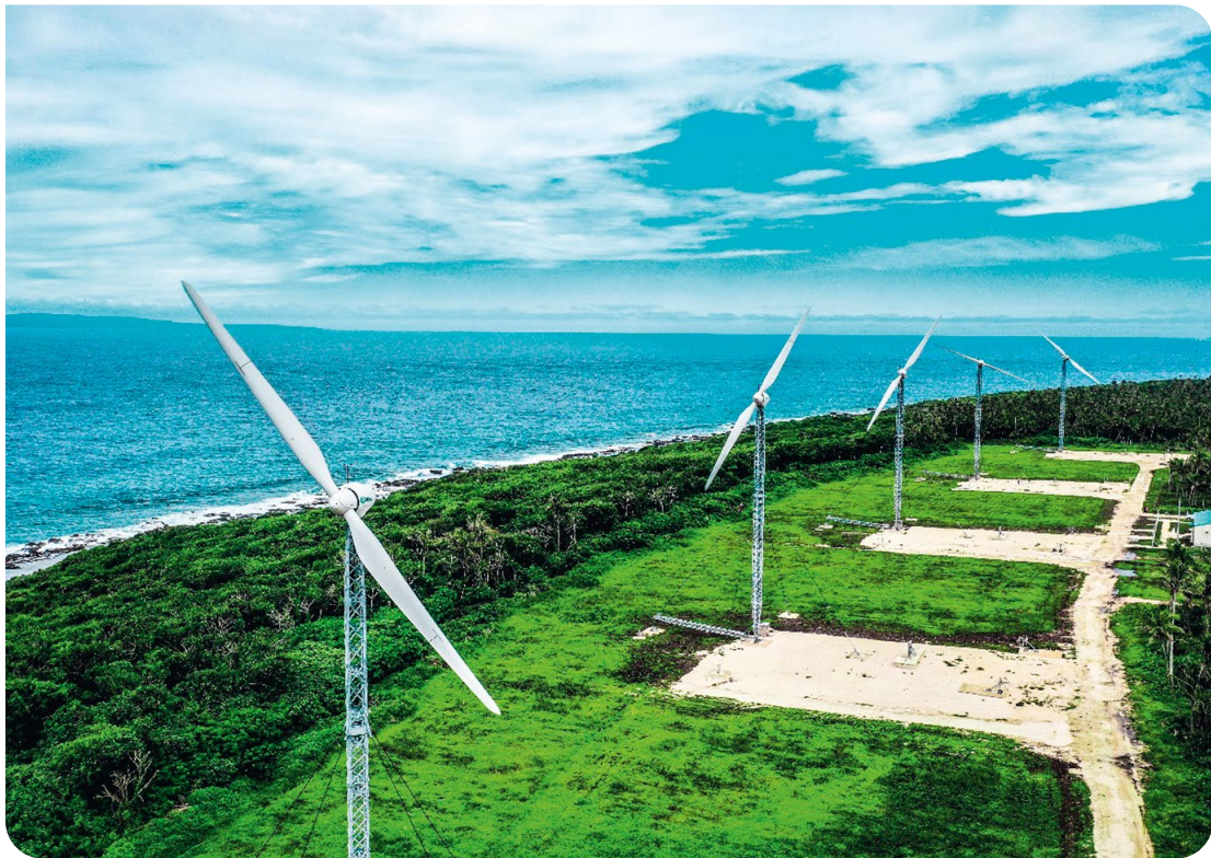
Tonga's first large-scale wind farm project, the Li'o Manumataongo wind farm, consists of five 275kW wind turbines.
