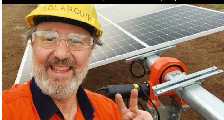
Installing a 70kW solar tracking system to power the Smart Energy Lab and seven homes connected to Glen Morris's microgrid at the community coop in the scenic hills east of Melbourne
