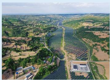
A Chinese 'Top Runner' PV power project in Tongchuan, Shaanxi, using 30MW TrinaPro smart solution.
